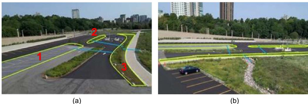
**Fig. 1.** Photo of green infrastructure facing north, with monitored infrastructure outlined in bright green (1: permeable pavers; 2: bioswale 1; 3: bioswale 2) and connectivity of the underdrains in blue (a); and photo of green infrastructure facing west, along with a gravel rip-rap channel that the system discharges into (b). (Images by Matthew Dupasquier.)
